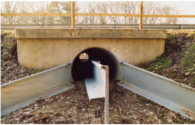
Corridors linking natural areas can include tunnels and bridges designed to enable wildlife movement. This “toad tunnel” under a German highway was built to be used by migrating amphibians. Christian Fischer/Creative Commons SA-3.0.
